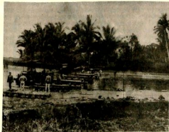
FIG. 2. BRIDGE ACROSS PIMI CREEK, AITAPE.
