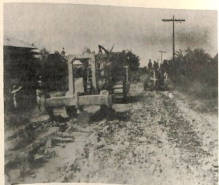
FIG. 21 RECONSTRUCTION OF HIGHWAY 7, DINALUPIHAN TO GUAGUA FOR ASPHALT SURFACE, CO. C.
