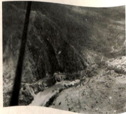
FIG. 29. AERIAL VIEW OF SLIDES 4 & 5, HIGHWAY 4, ALONG IBULAO RIVER.
