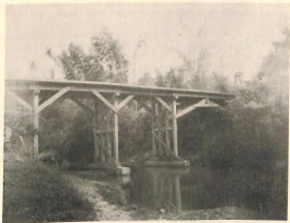
FIG. 24. CATMON RIVER BRIDGE, 120' LONG, NORTH OF SANTA MARIA, BULACAN, CO. A.
