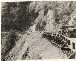
FIG. 31. BRIDGING SLIDE 5, HIGHWAY 4, CO. B.
