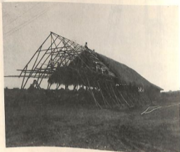
FIG. 25. THEATRE BUILDING, SAN ILDEFONSO AREA.
