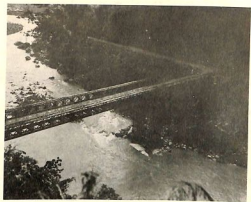
FIG. 33. IBULAO RIVER BAILEY BRIDGE, HIGHWAY 4, COS. A & B.
