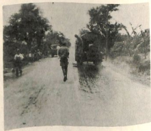
FIG. 22 ASPHALT DISTRIBUTOR IN OPERATION, CO. C.
