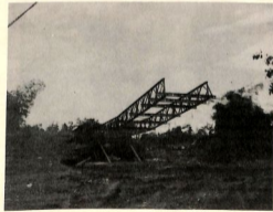
FIG. 20. 280 FT. DOUBLE-DOUBLE BAILEY, SANTA MARIA RIVER, IPO ROAD, CO. A.
