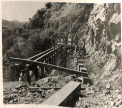
FIG. 28. BRIDGING SLIDE 1, HIGHWAY 4, NORTH OF BAGABAG, CO. B.
