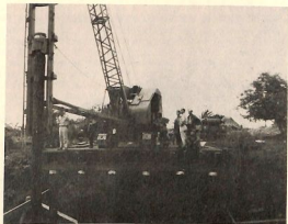
FIG. 23. DRIVING PILING, ROUTE 5, SABANG, BULACAN CO. C.
