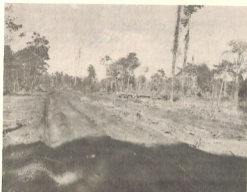
FIG. 4. ROAD CONSTRUCTION AT TOEM, D.N.G.
